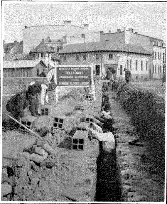
Underground Conduit Work in Progress in Bucharest.
