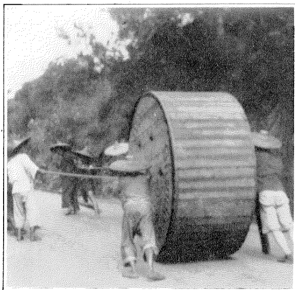
Figure 8—Distributing Drums Along Road in British Territory.
