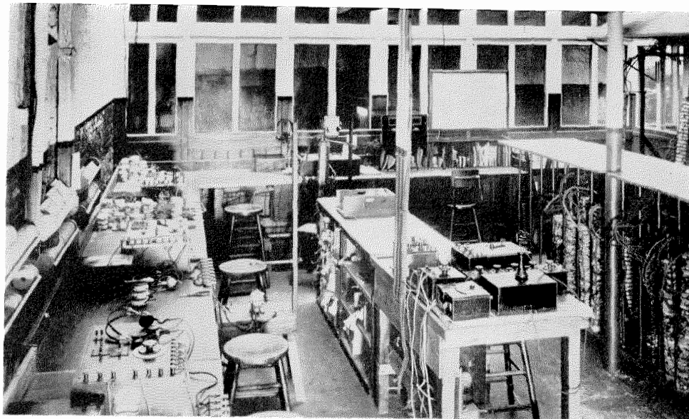
Figure 22—Dowel Assembly and Test Room.
